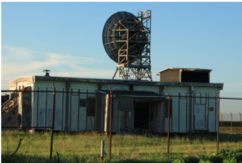
Former DEW Line training facility, Streator, IL. National TLC Photo.
